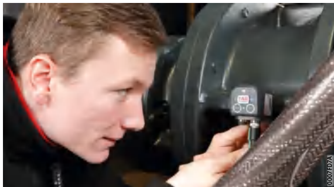
Figure 3 Commissioning of FAG SmartCheck
